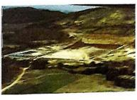
it to the smallest practical volume; heavy tractor-like equipment is used to spread, compact and cover the waste daily, usually with at least six inches of compacted soil or other fill meterial. After the area has been completely filled and covered with a final two to three foot layer of soil, it is allowed to settled for an appropriate period of time.
